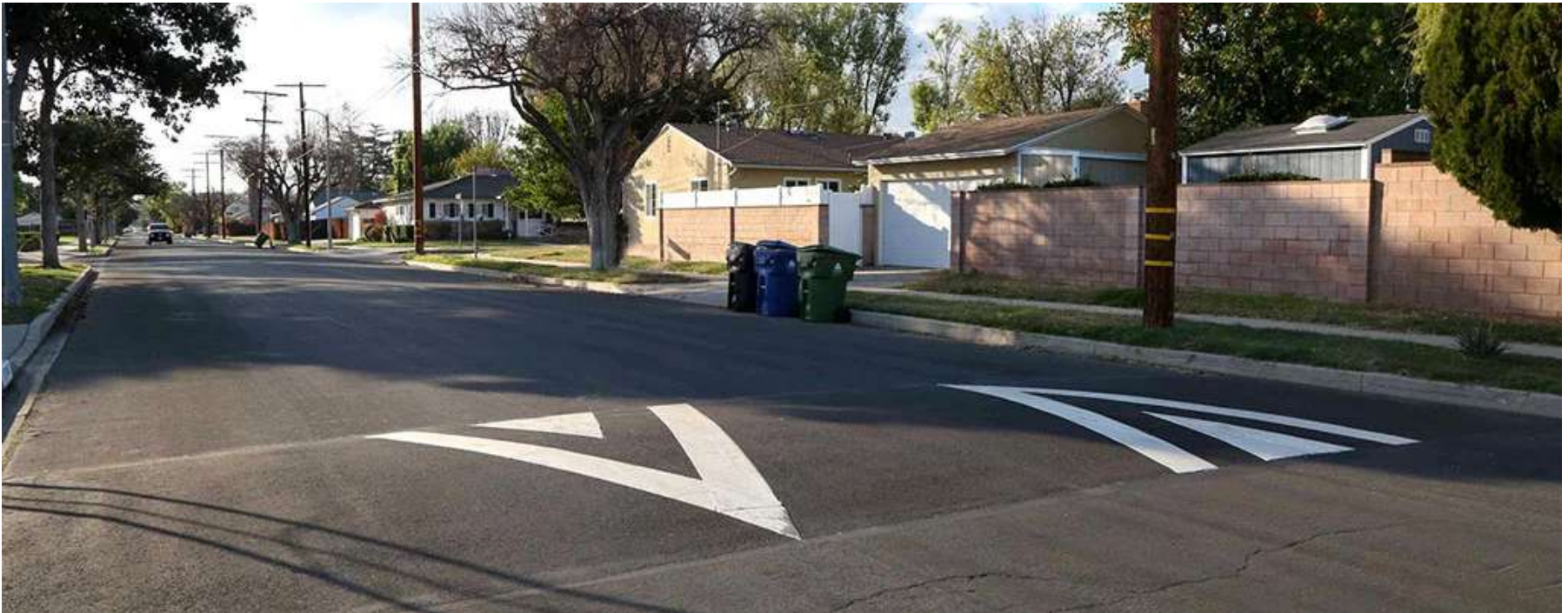
Image Caption: Speed Hump and Accompanying Warning Markings
