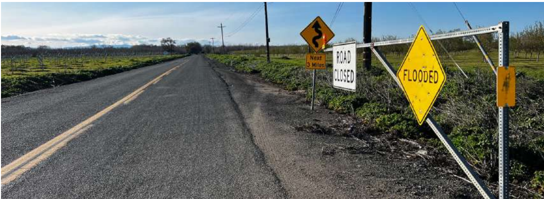
Image Caption: Example Flood Closure Gate
