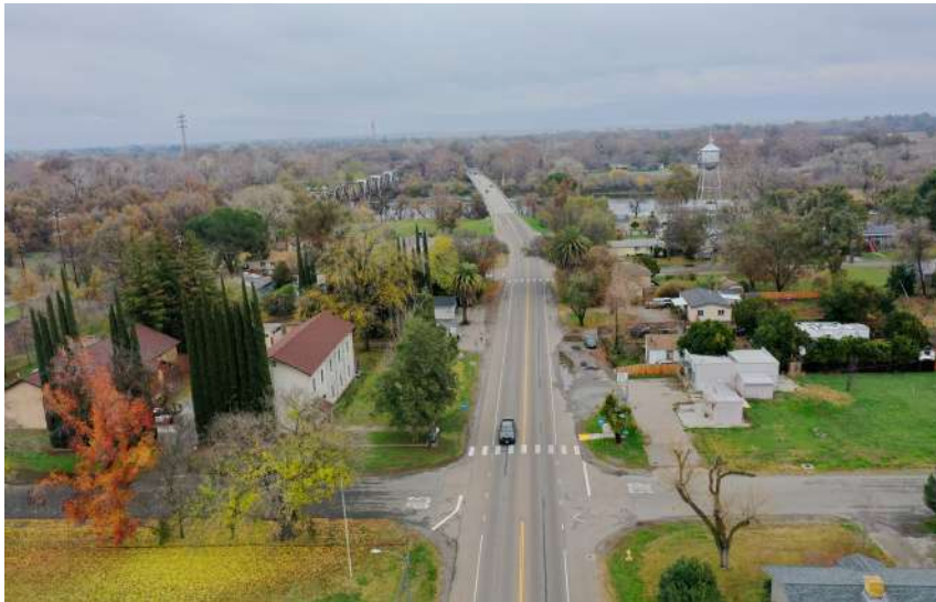
Image Caption: C Street from Above, Facing East
